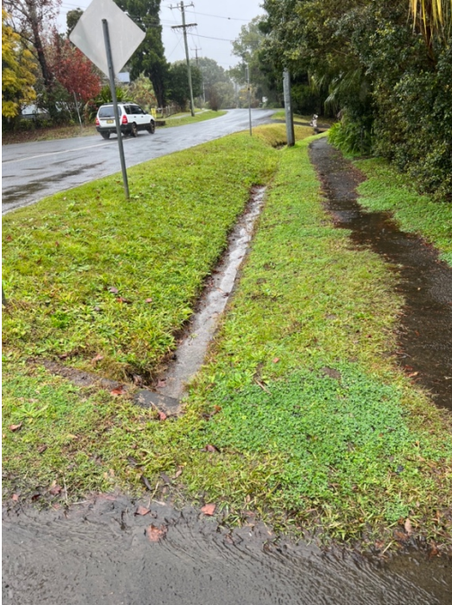
Drainage works well until it meets a blocked drain – then the footpath becomes a rivulet
